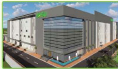
UPCOMING MANUFACTURING UNIT - 3
